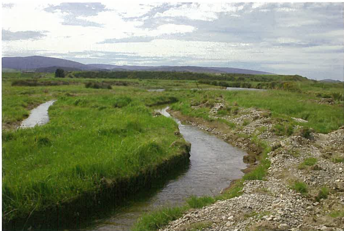
Above and below: Whitebait Project. In spring 2013, the permanent low gradient/low velocity outlet channel between the McCulloch Wetlands and the Waiiau Lagoon, was under construction. Holly Burn mouth behind digger. The 400m meandering channel provides crucial fish passage for all upstream and downstream migrating fish, particularly Inanga.
