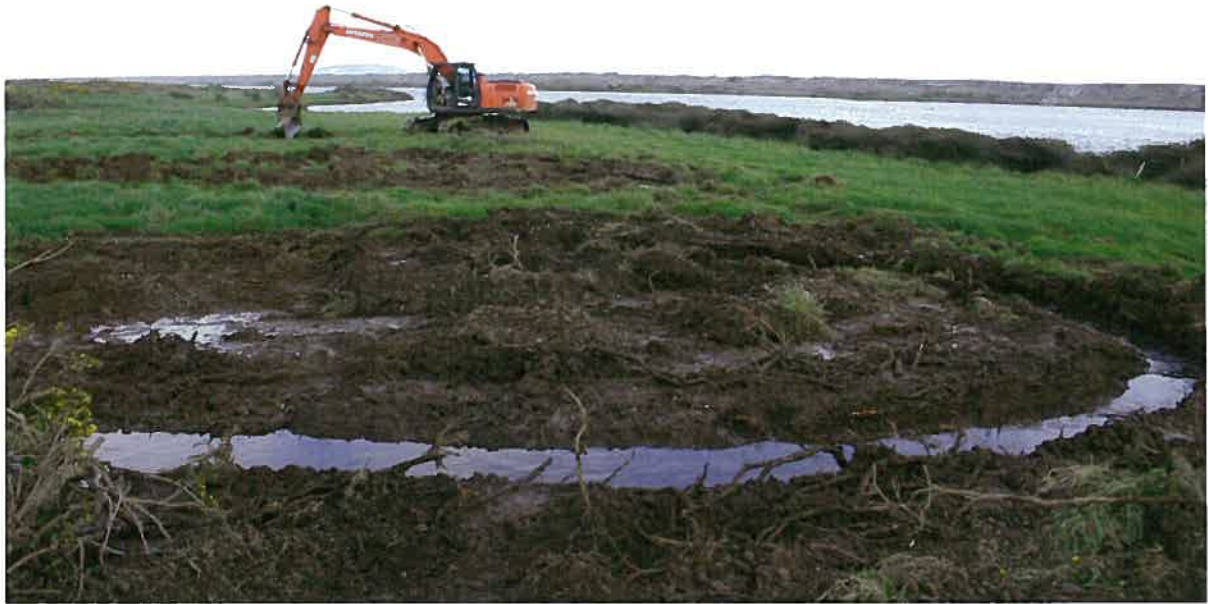
Above and below: Whitebait Project. In spring 2013, the permanent low gradient/low velocity outlet channel between the McCulloch Wetlands and the Waiiau Lagoon, was under construction. Holly Burn mouth behind digger. The 400m meandering channel provides crucial fish passage for all upstream and downstream migrating fish, particularly Inanga.
