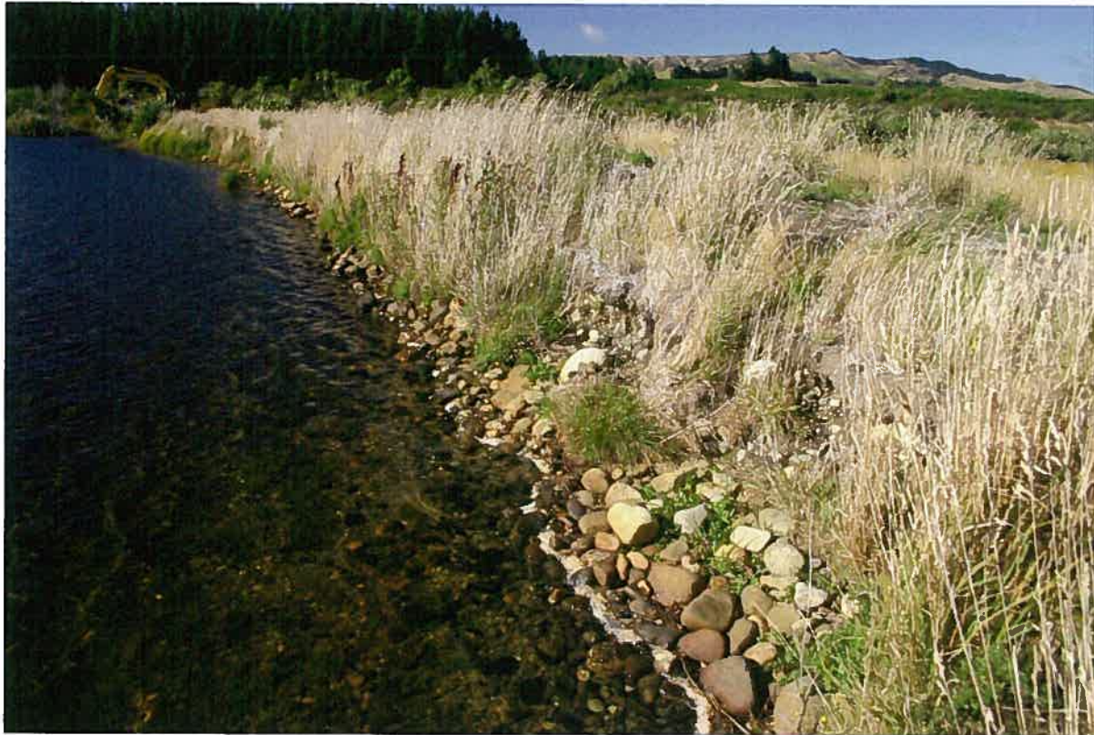
Rakatu Wetlands April 2013: The lower Rakatu dam has suffered some wave lap damage over the past 8 years (above). This was repaired by strategically placing flax and other vegetative material along the face of the dam to act as a natural buffer. Below , the job nearing completion.
