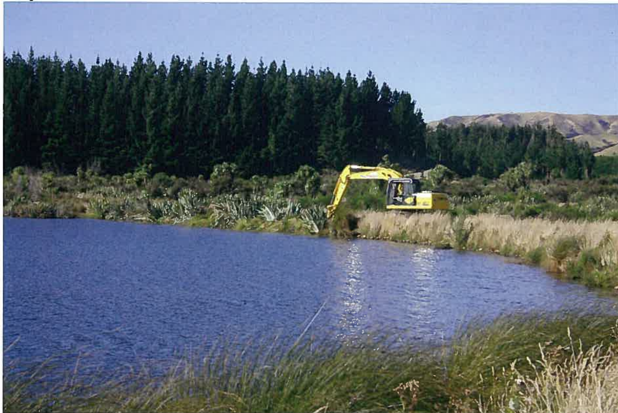
Rakatu Wetlands April 2013: The lower Rakatu dam has suffered some wave lap damage over the past 8 years (above). This was repaired by strategically placing flax and other vegetative material along the face of the dam to act as a natural buffer. Below , the job nearing completion.
