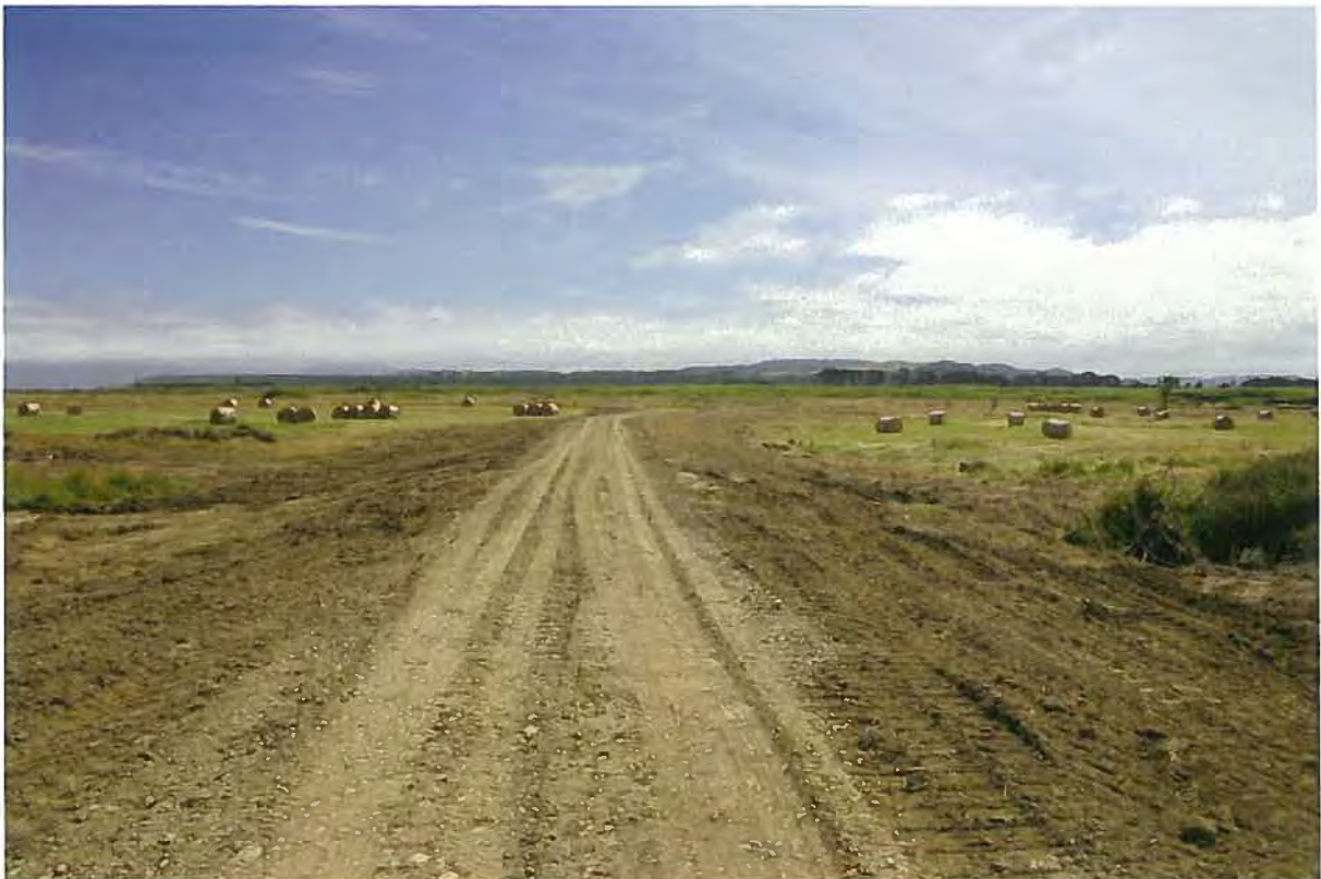
The completed dam with topsoil on the batters and the crest, ready for seeding. The dam has 500mm of freeboard and 6:1 batters.
