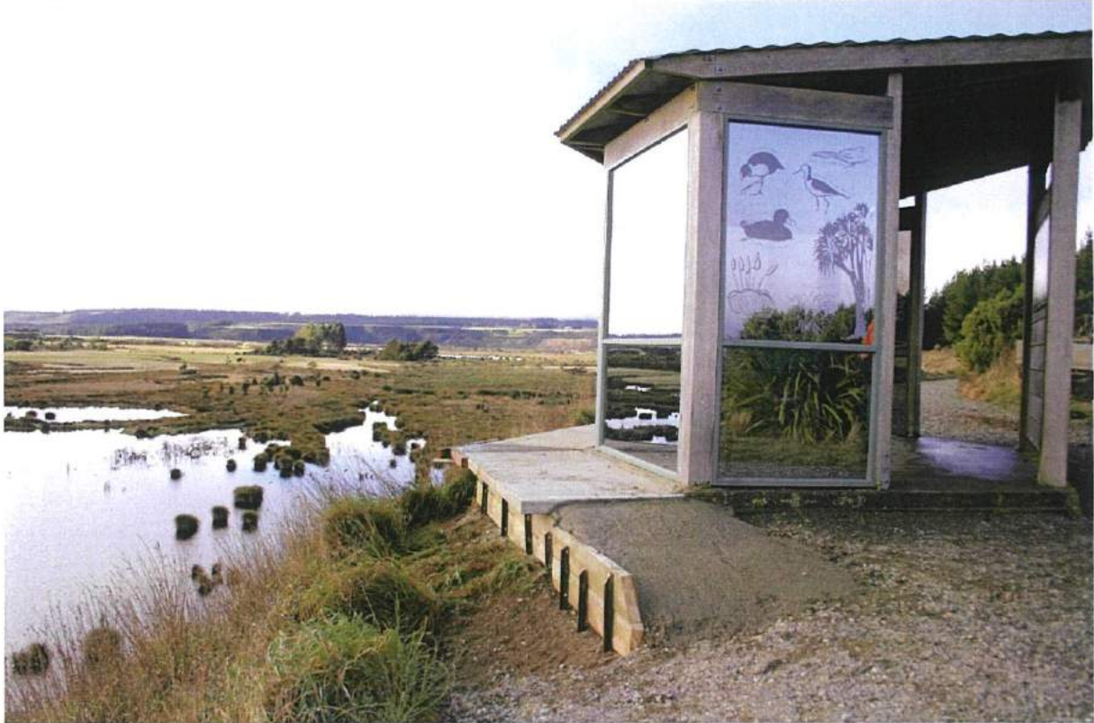
Lookout structure above Speights Stream 1 wetland: Concrete reinforcing was installed at the front of the structure, as part of the normal maintenance programme at this site.
